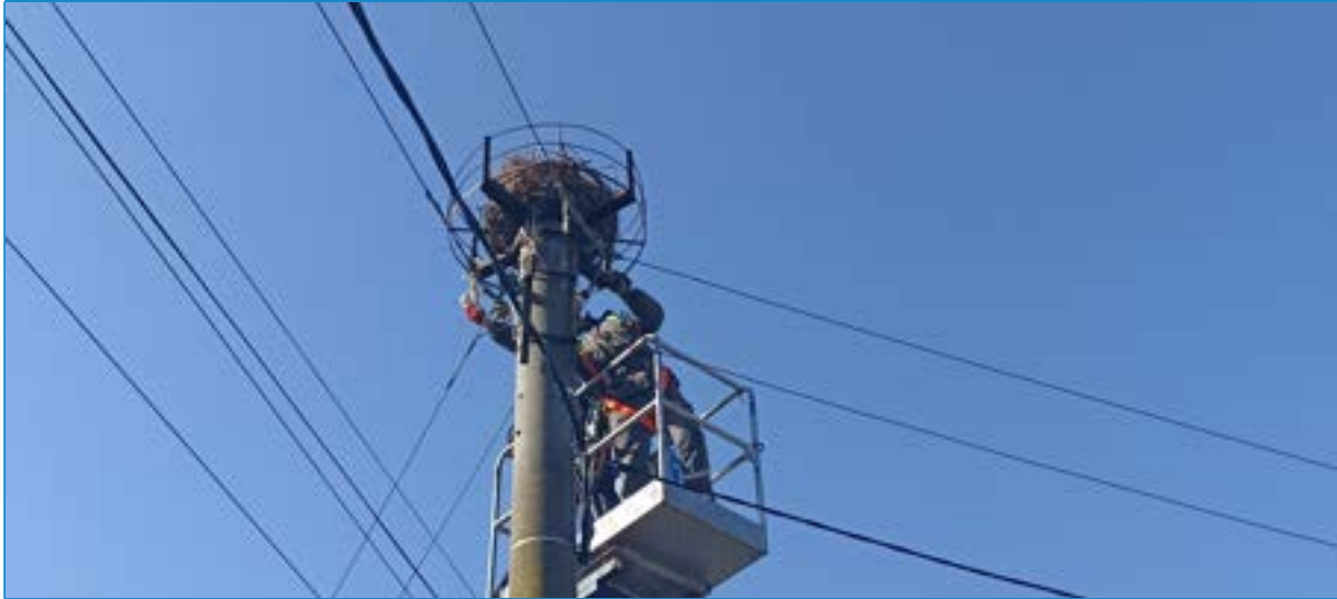
Picture 1: Bulgaria team conducting periodic inspections
